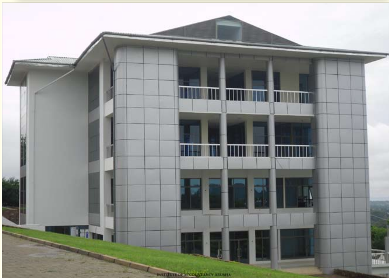
Institute of Accountancy Arusha New Library Building
